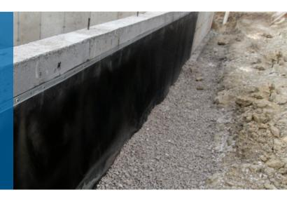
If something is engineered to keep liquids in, it only makes sense that it would do a good job of keeping them out. Plastatech® IG (Industrial Grade) and Plastatech Tech 5® geomembranes are popular solutions for basement wall and foundation waterproofing in commercial and industrial applications. Plastatech geomembranes provide a highly effective barrier to water intrusion in any climate.
