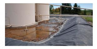
Our geomembranes are specially formulated to remain highly flexible and resistant to cracking or puncture on rough or uneven surfaces — even across the entire range of normal operating temperatures. They can also be formulated to be highly resistant to degradation from ultraviolet light, making them suitable for a wide range of applications which are exposed to the elements.
