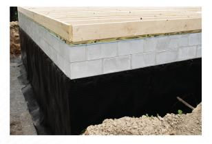
Their flexibility and puncture-and-tear resistance allows them to be installed against concrete, block and even old brick foundations — while avoiding punctures and tears during backfill. Their flexibility in high and low temperatures allows them to provide years of trouble-free use.
