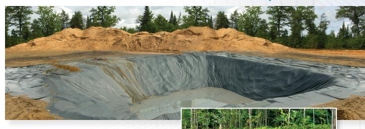
Geomembranes are used for a variety of applications, from containing potable water to lining landfills and ponds. The best material for the job depends, to some degree, on the specific application.
